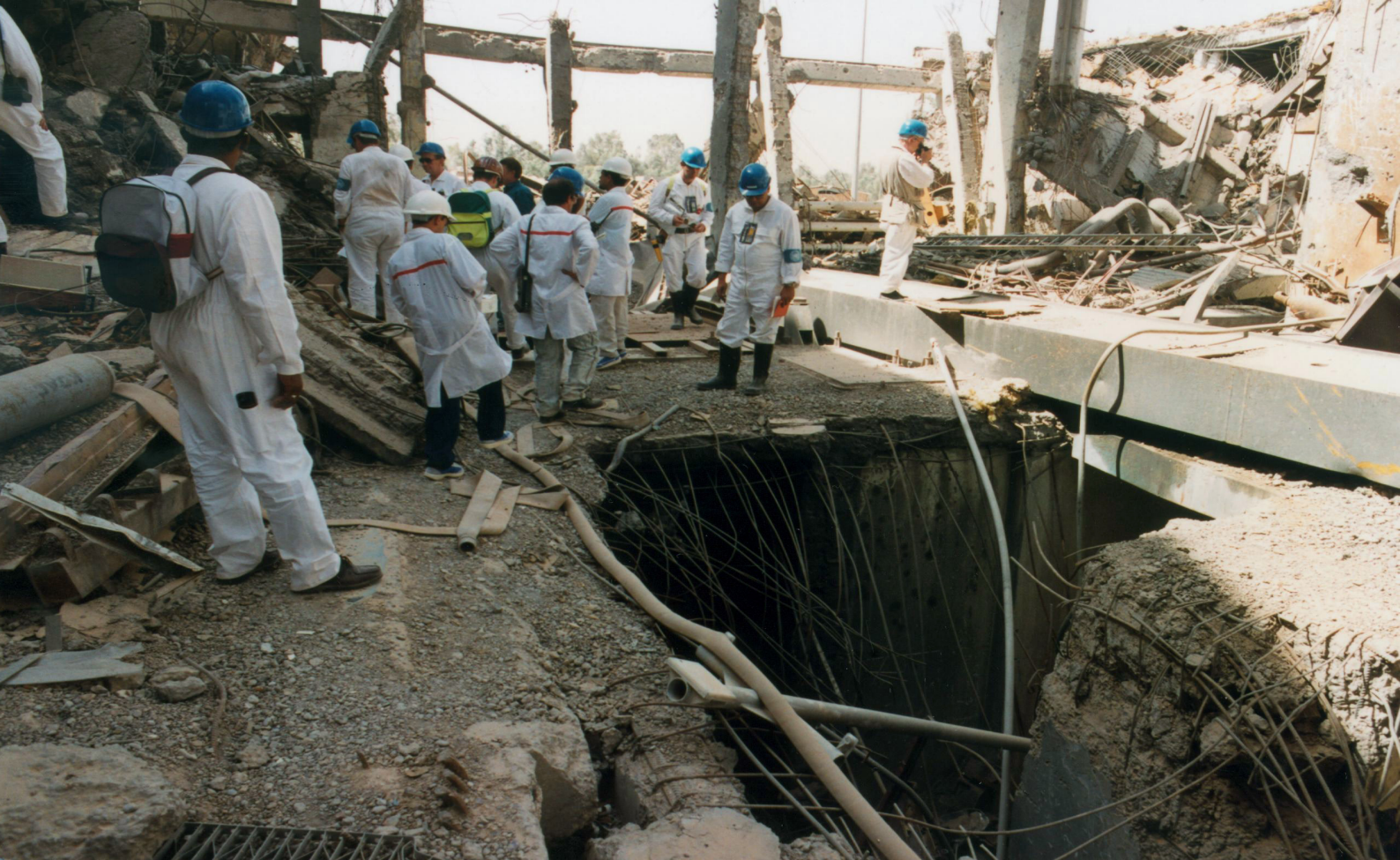
Inspectors visit the ruins of a facility used to produce highly enriched uranium for Iraq's nuclear weapons program. Photo Credit: Action Team 1991-1998/IAEA.
