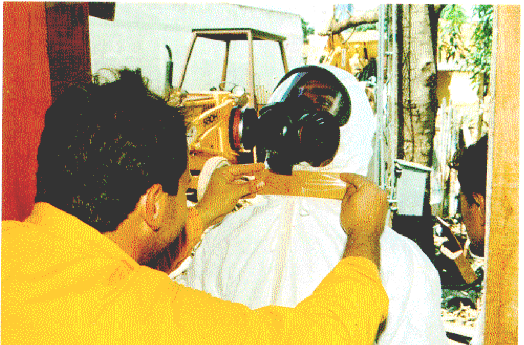
Preparing to demolish the contaminated houses
