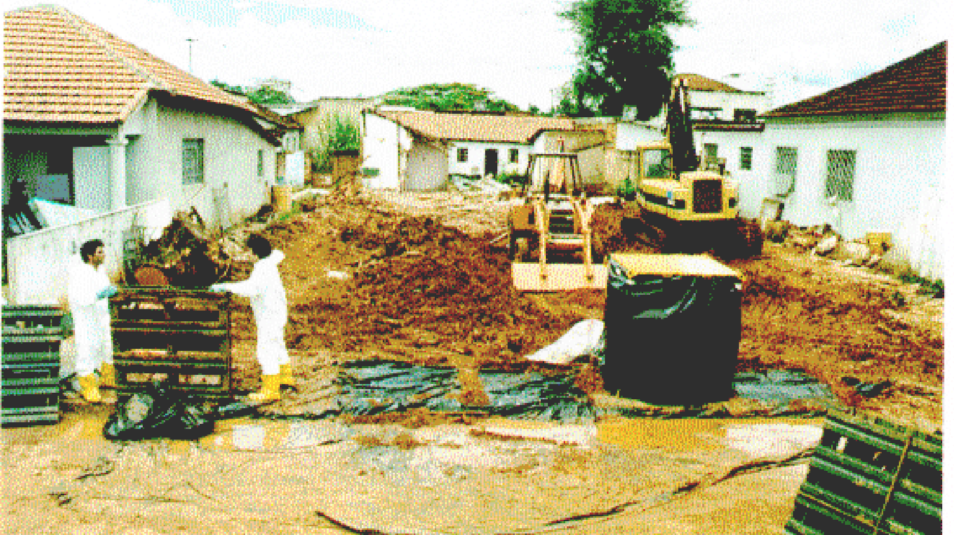
Restoration after removing the contaminated rubble
